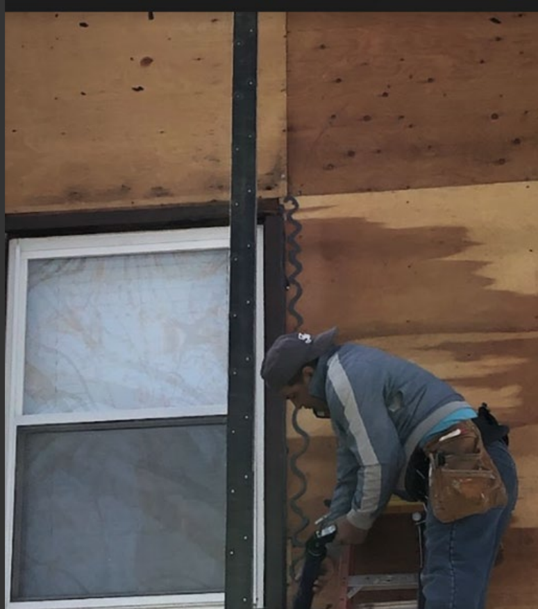
Liquid flashing application at window jamb
