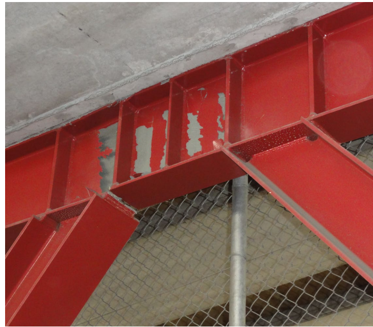
Eccentrically Braced Frame with damage in the Link Beam (Christchurch, NZ 2011)
