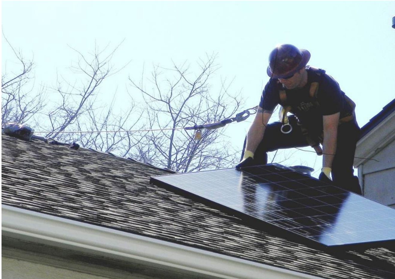
Fall exposures during solar panel installation Photo: California Department of Public Health
